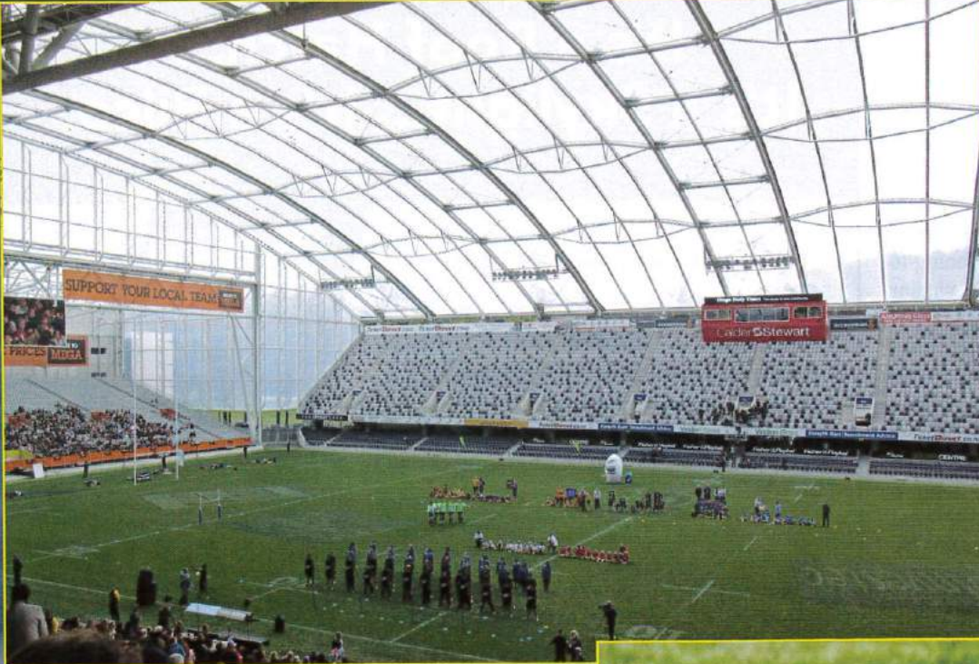
Figure 11 - ETFE roof spanning the playing field.
