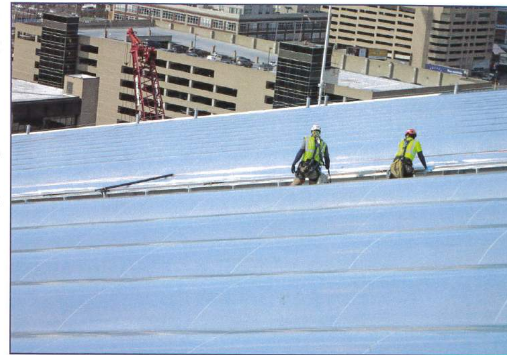
Figure 20 – Installation of ETFE cushions.
