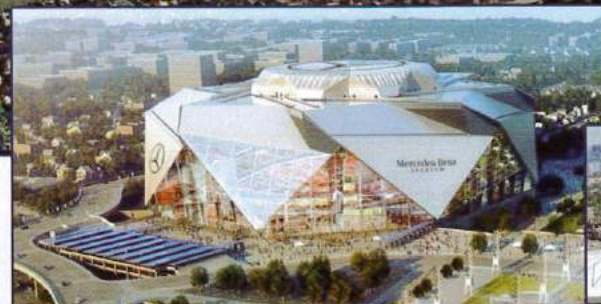
Figure 22 - Rendering of the Mercedes Benz Stadium showing ETFE roof system and ETFE cladding system. Photo by HOK.
