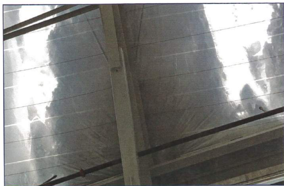
Figure 10 – An ETFE system in a deflated state, supported by snow cables, with snow load. Photo by SurfaceDesign.
