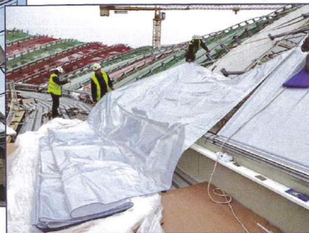
Figure 15 – Installation of ETFE cushion. Photo by Birdair.
