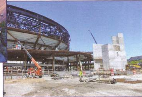
Figure 25 - Current construction of arena and surrounding structures.
