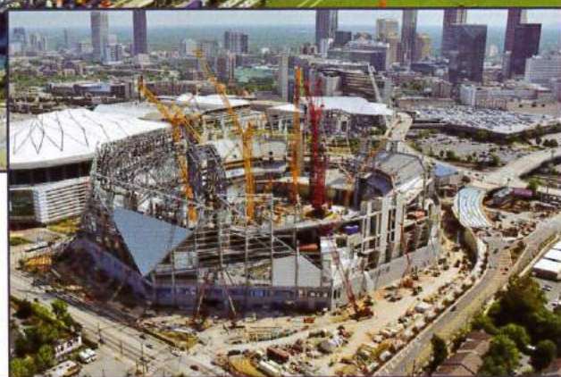
Figure 23 - Current construction of stadium. Photo by www.11Alive.com.
