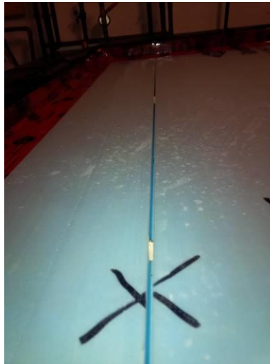
Figure 6 – Insulation Board Gaps
