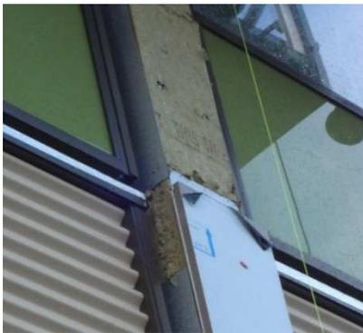
An example where the assembly U-values might be fine when thinking in parallel but the overall thermal performance is poor because of thermal bridging at interface details
